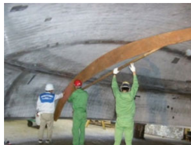
Figure 5.2 Dimension check of vessel head inside
