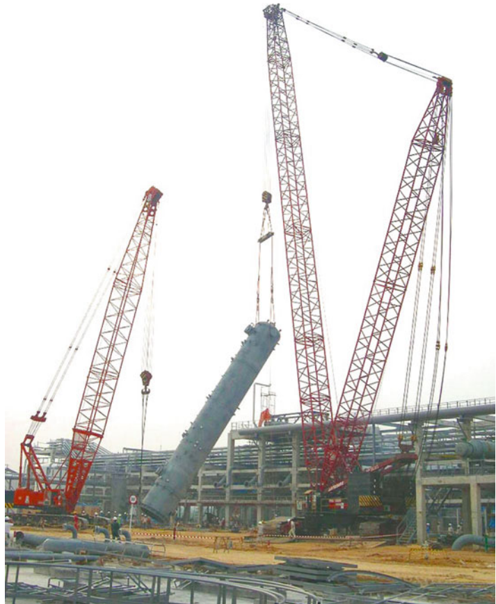
Figure 3.6 Erection of Tall Pressure Vessel-Posted by Richard L. Krabbendam. (Source: http://www.heavyliftspecialist.com )
