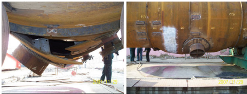
Figure 5.34 Failure during hydrotest in pressure vessel manufacturing shop
