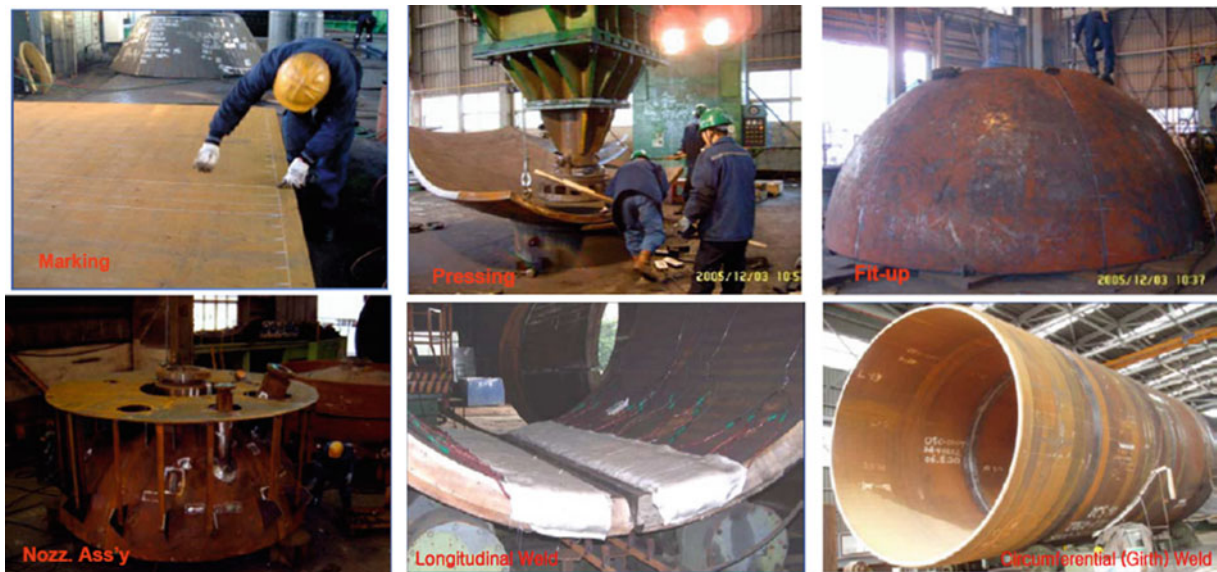
Figure 3.1 Major Steps of Pressure Vessel Fabrication
