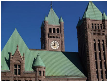
Figure 2.90 Copper roof on the Minneapolis City Hall, coated with patina. (Source: Wikipedia)
